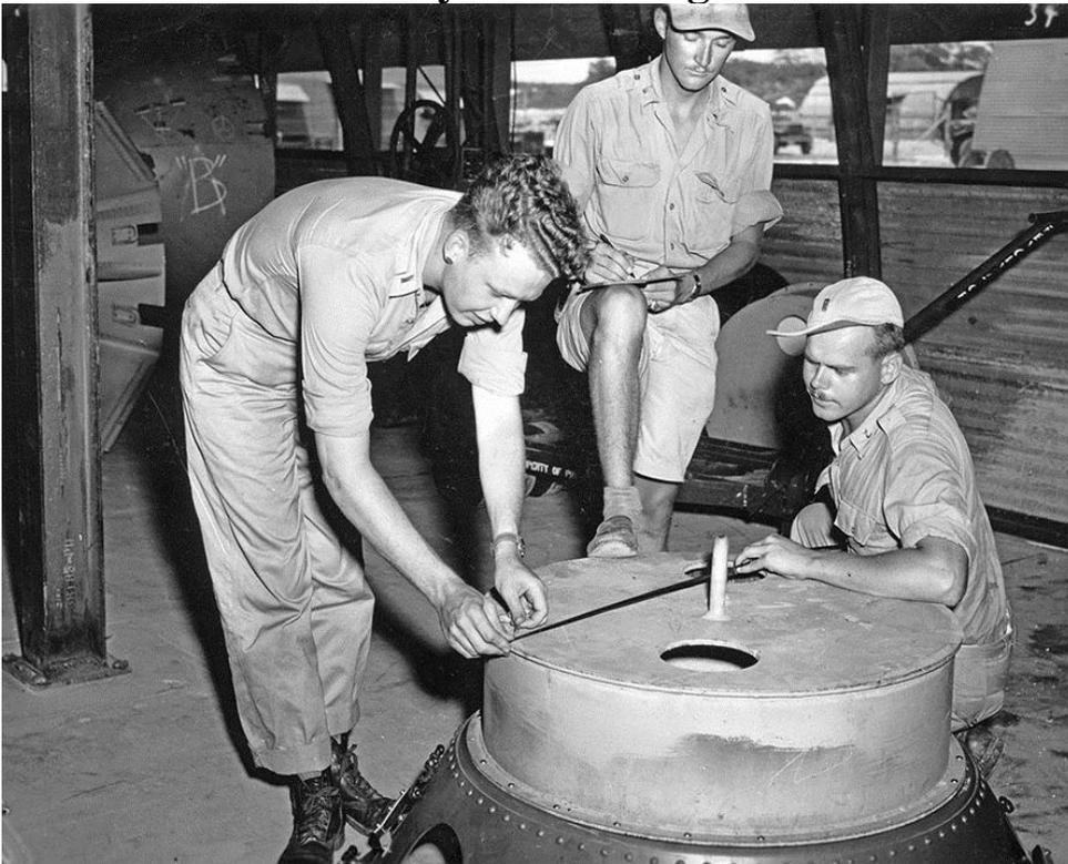
**Photograph of personnel checking a casing.** A significant number of extra casings were shipped to Tinian and used in various tests with “dummy” bombs, which contained all the active components of a working atomic bomb, but no fissile material to test out and prove the assembly procedures for the actual devices themselves.
