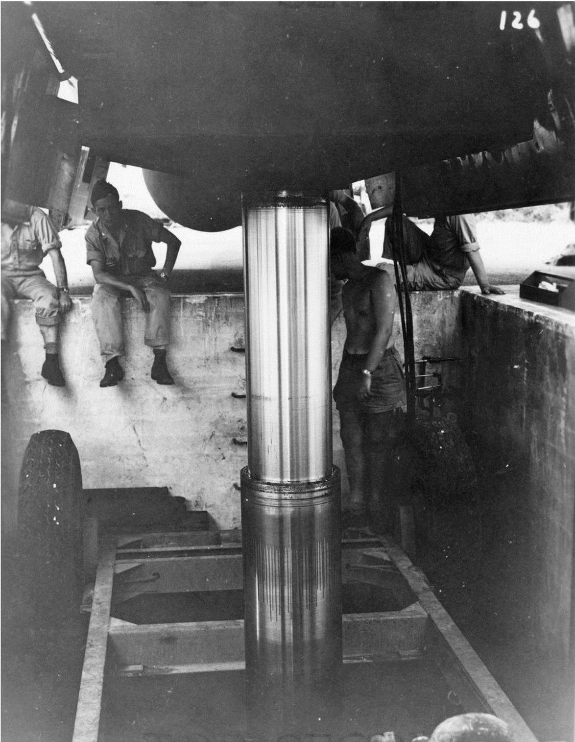
**View from within the pit showing the dolley frame and the fully extended hydraulic lift.**
