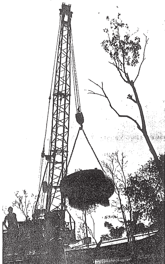
BIG LIFT -- Relocation of the 4th Division's base camp necessitated the installation of several additional water tanks at Camp Radcliff.
